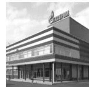
СК «Газпром Прометей» Construction Company "Gazprom Prometheus"
